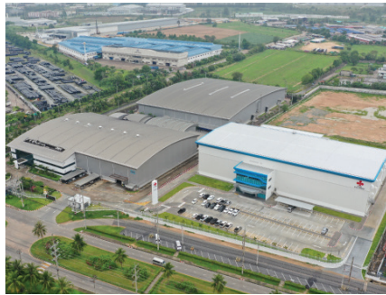
Rayong Plant - Cleanroom
